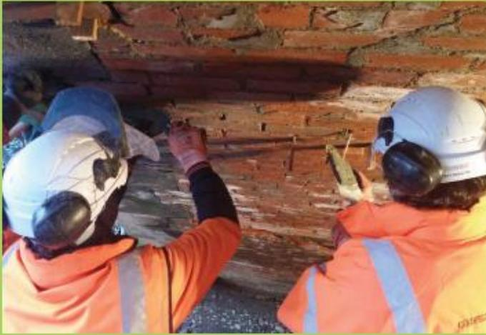
The Goldfield Stone team, placing mortar around newly installed bricks
