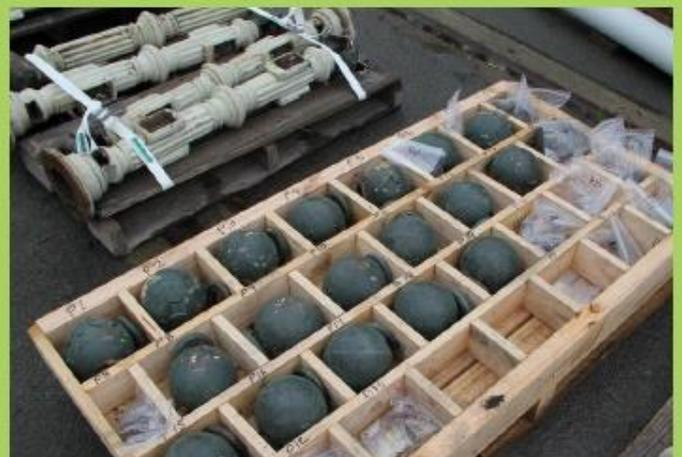
A built for purpose storage box for the dismantling of balustrade. Each compartment was labelled to ensure it was returned to the correct place
