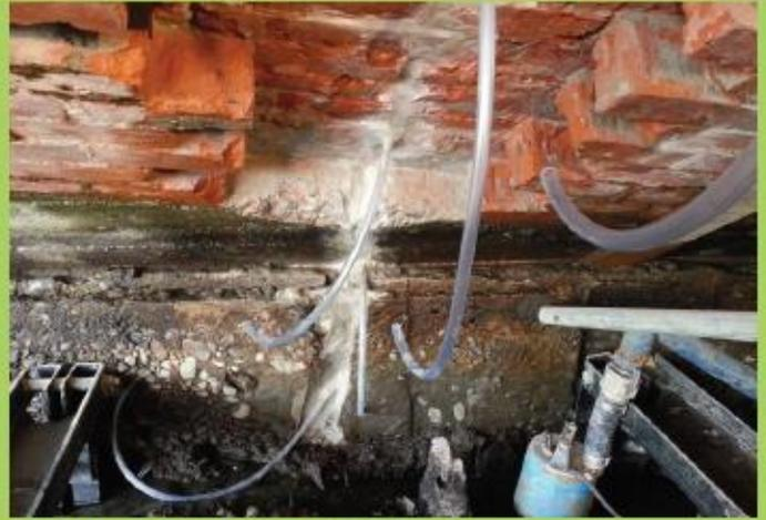
Installation of grout tubes ready for injection
