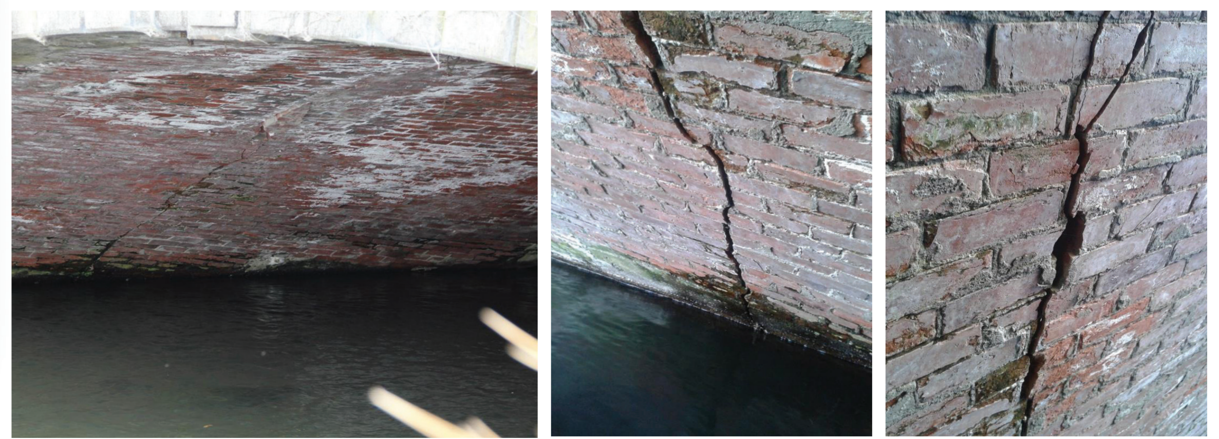
Images show cracking to the brickwork beneath the Armagh Street bridge.
