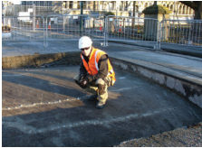
Site engineer Tom Harding-Ilott checks the repaired, resin-filled cracks running across the top of the brick arched bridge.
