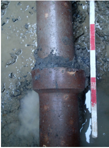
Part of a 100mm diameter earthenware pipe drain private sewer connection installed c. 1885, St Asaph Street. Individual pipes were joined together with a coal tar type material rather than a rigid cement mortar.
