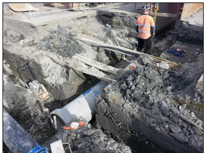
Criss-cross: Utilities cross over a new pipe at the intersection of Edgware Road and Colombo Street in Christchurch.
