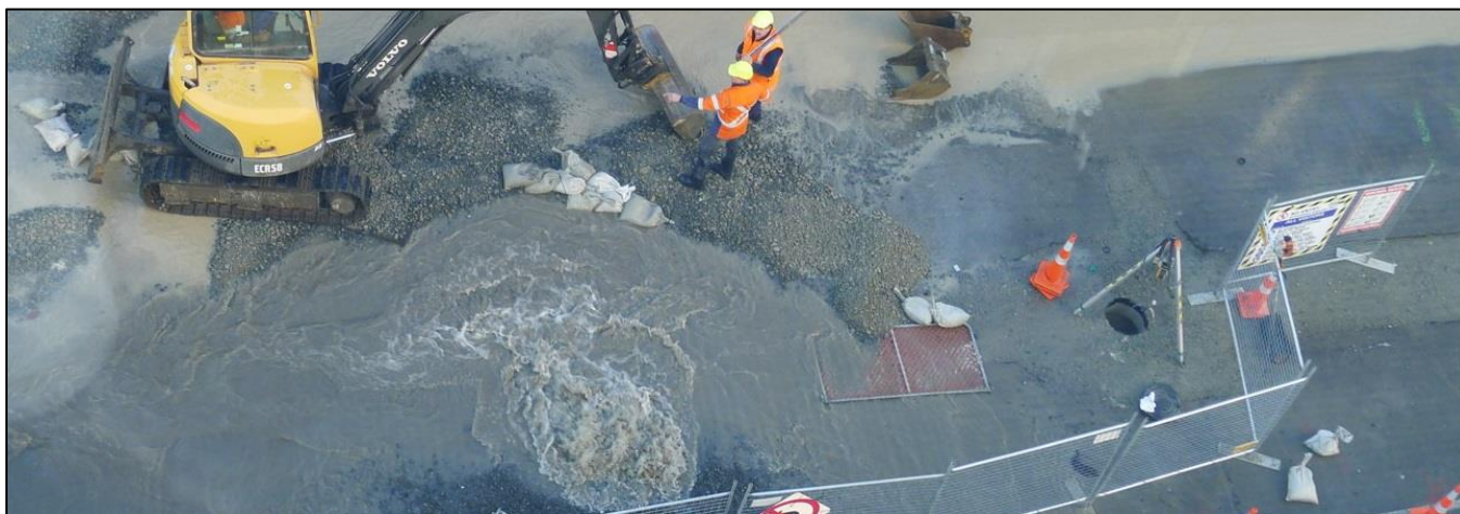
High water: A water main strike in Gloucester Street, central Christchurch.
