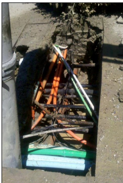
Spaghetti junction: A jumble of underground services on Edgeware Road, Christchurch.
