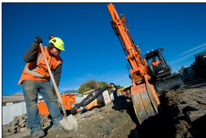
Easy to spot: A “spotter”, wearing personal protective equipment (PPE), looks out for underground services.
