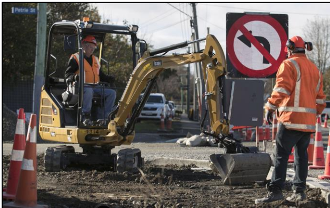
Got your back: A “spotter” guides an excavator operator as the road surface is scraped in Petrie Street, Richmond.
