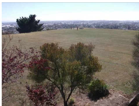
Figure 1: Huntsbury No.1 Reservoir. Christchurch's largest reservoir (capacity 35,000 m 3 ).
