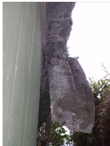
Figure 7: Clifton 3 – internal column failure.
