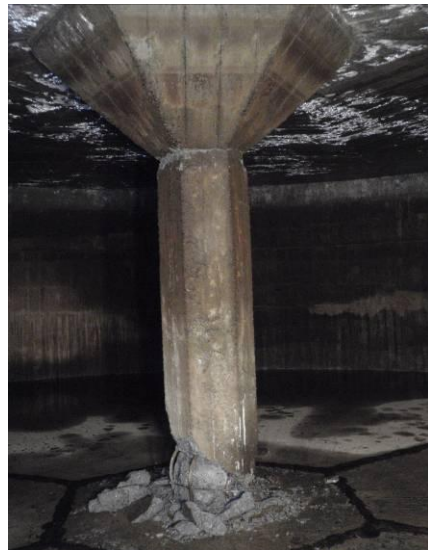
Figure 7: Clifton 3 – internal column failure.
