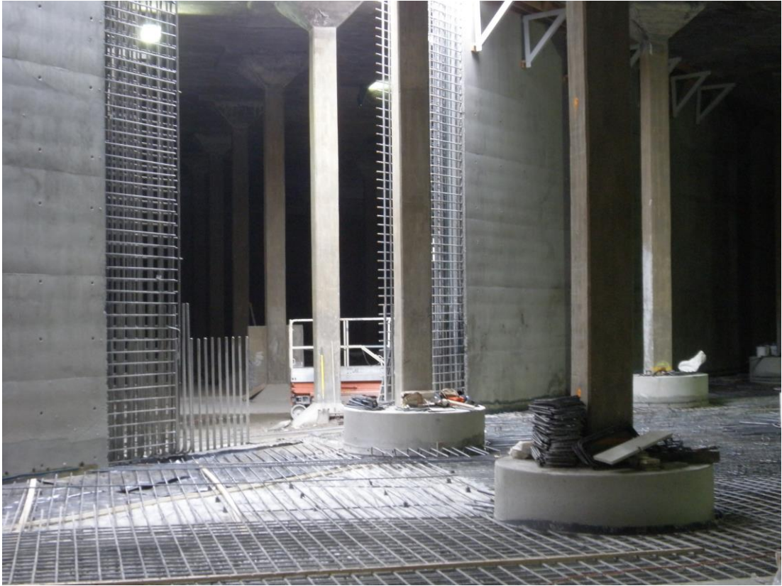
Figure 5: New Floor and Wall Sections under construction
