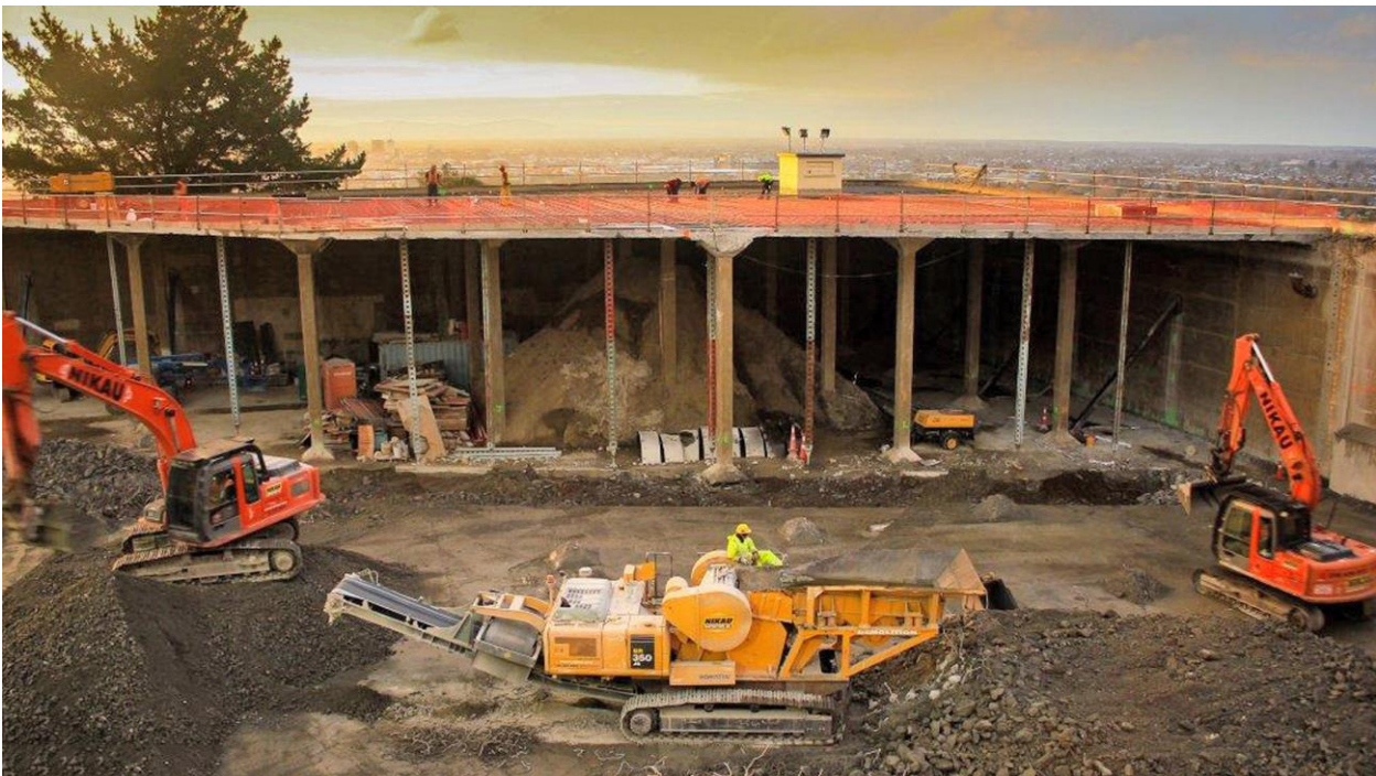
Figure 2: Huntsbury No 1 stage 2 reservoir - under construction
