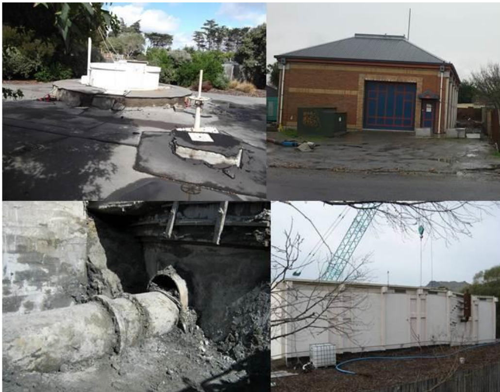
Photograph 9: Pump Station Earthquake Damage
