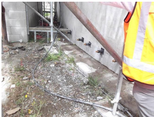
Photograph 7: McCormack's Bay Shear Connection Wall to Floor
