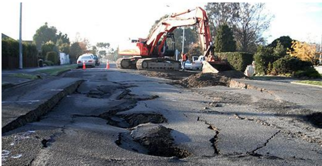
Photograph 12: Woodham Road Trunk Main Failure
