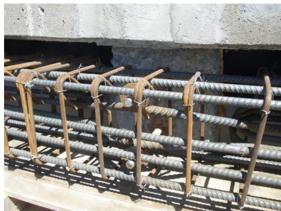
Photograph 5: Upper Balmoral Reservoir Ring Beam Reinforcing
