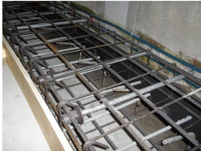
Photograph 8: Shear Connection Wall to Floor Slab
