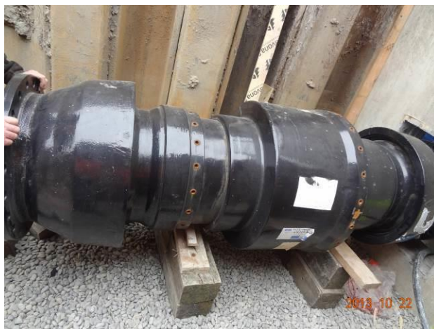
Photograph 10: EBAA Flex-tend Fitting (PS105)
