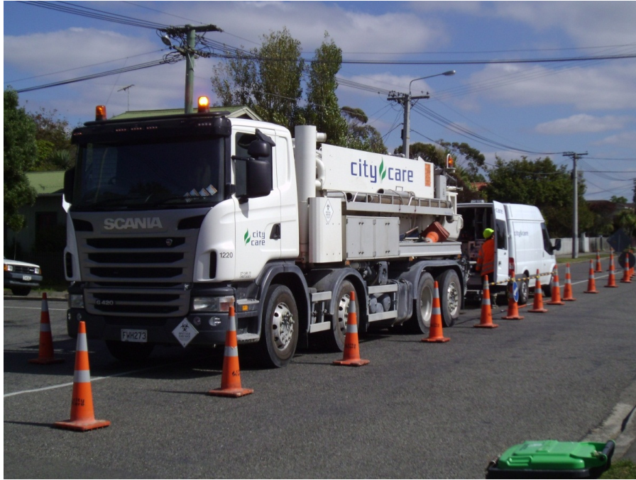
Figure 1: Typical CCTV Operation with combined jetter/sucker truck and CCTV Van
