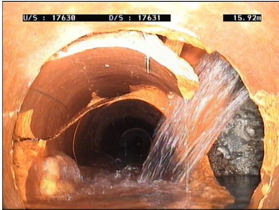
Figure 3: Breaks in EW pipe resulting in Tono
