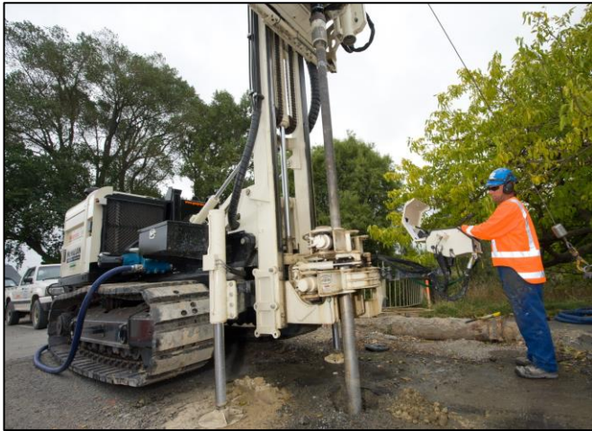
Sonic dig: A worker uses a sonic rig to cut boreholes to test ground conditions in Fitzgerald Avenue.
