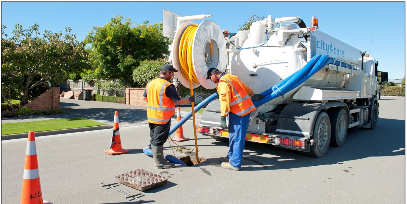
Time for a close-up: Work crews use CCTV to check for underground damage.
