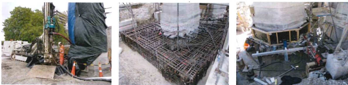
Figure 6. (L-R) Pilling Work, Pile Cap Reinforcement, Rocking Collar Coring
