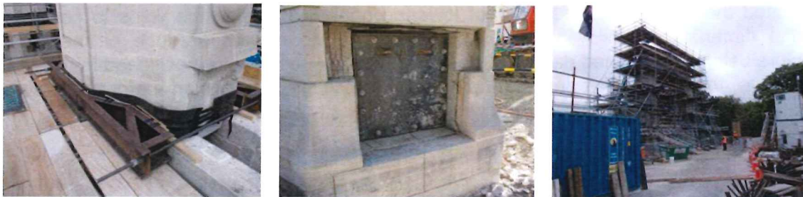
Figure 4. (L-R) Steel Column Clamp, Temporary Access Hatch in side of Column, Scaffolding
