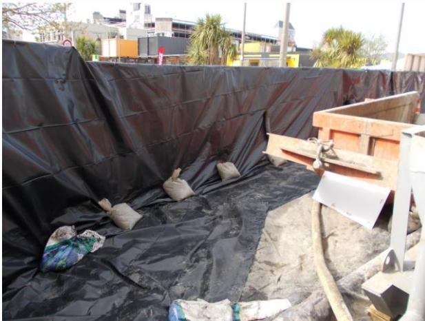
Black Plastic attached to Site Fencing
