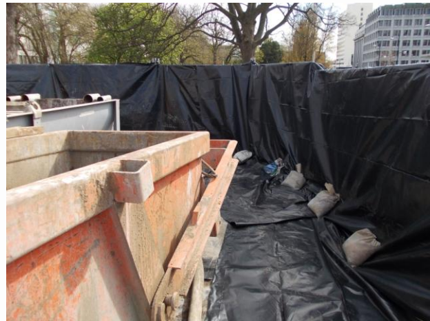
Black Plastic attached to Site Fencing
