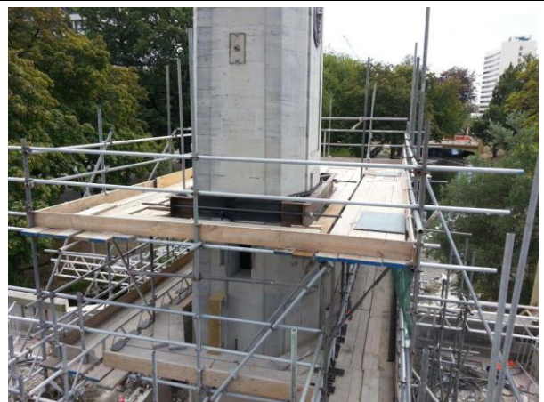
Seismic Clamp Installed
