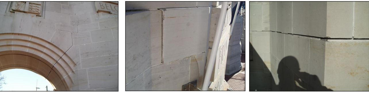
Figure 1: Crack map and typical cracks recorded after the February 2011 Earthquake
