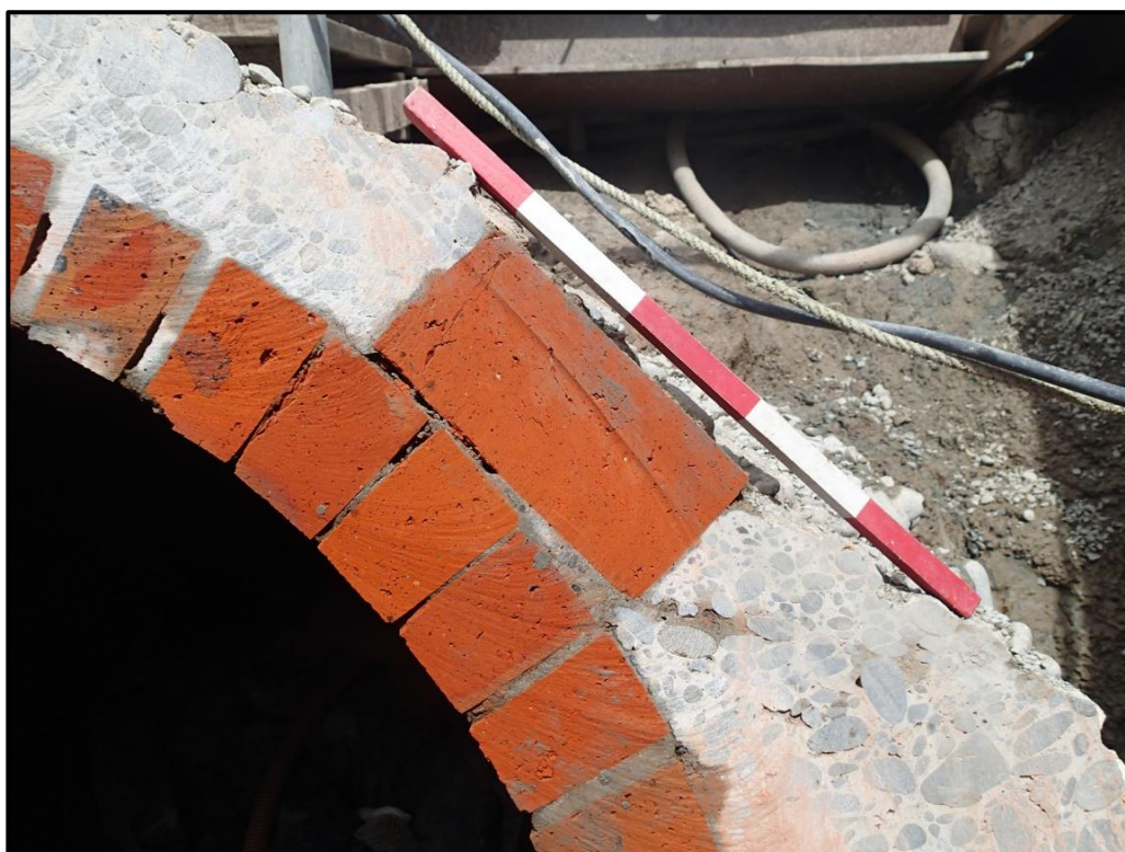
Figure 18. Section of the upper crown of the brick barrel. Note the rounded aggregate in the concrete, and the brick incorporated as aggregate.
