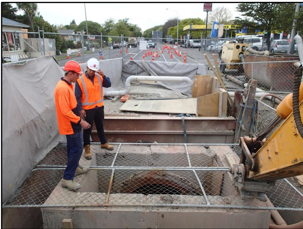
Figure 5. Looking east along Ferry Road, with the completed manhole atop the brick barrel in the foreground.
