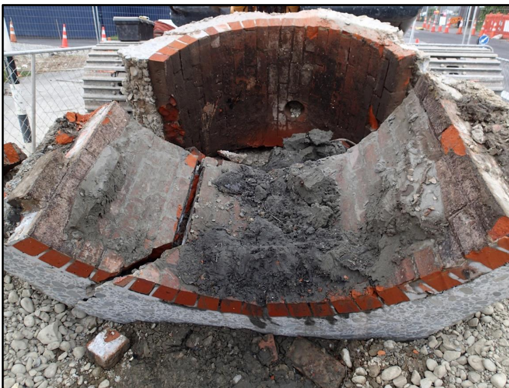
Figure 7. The removed section of brick barrel.
