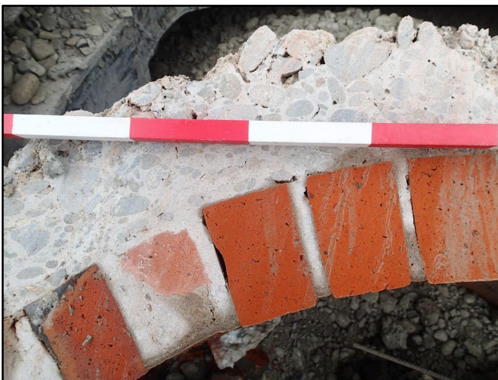
Figure 8. A section of the upper crown of the brick barrel, showing the arrangement of bricks haunched in concrete.
