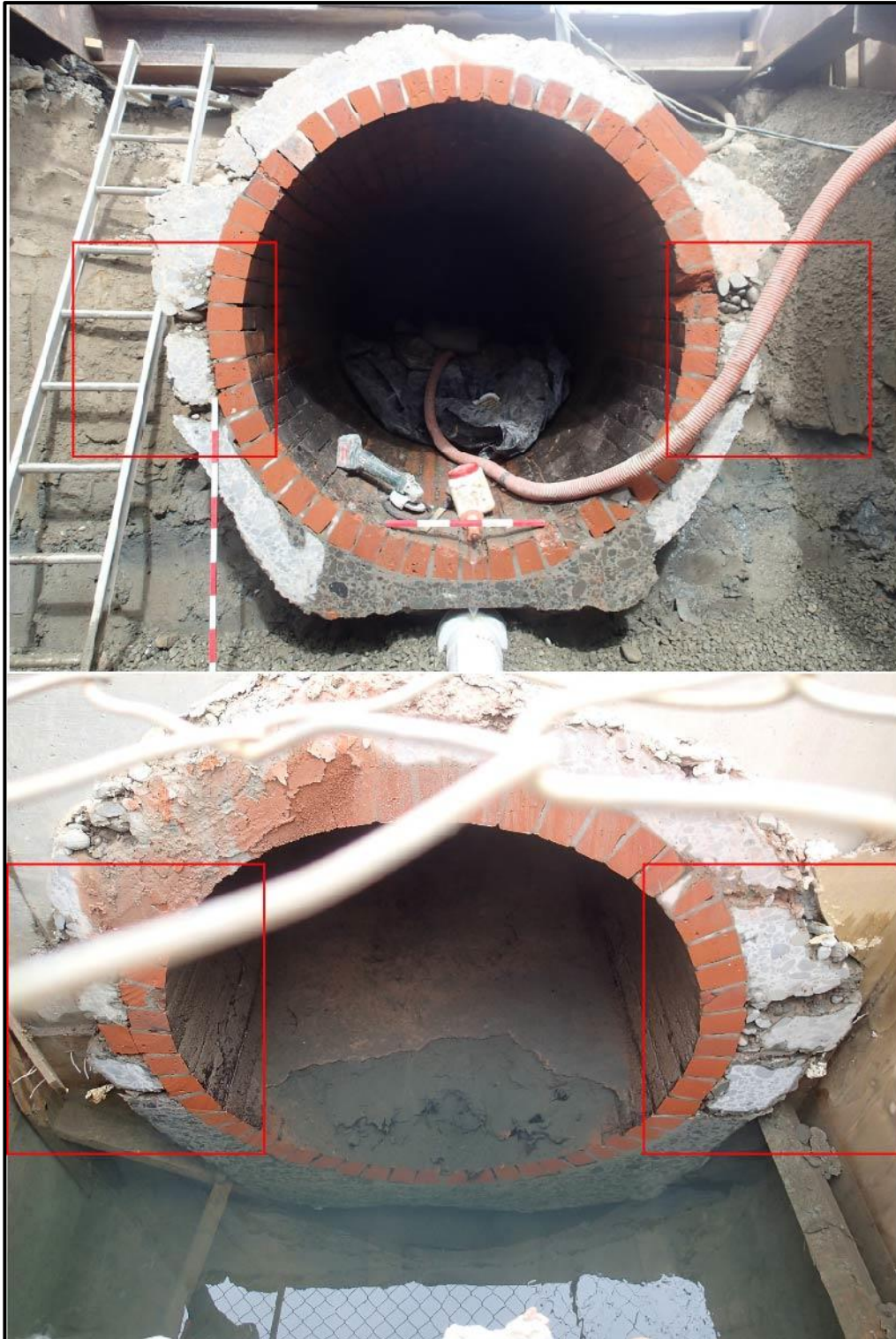
Figure 20. At top, the Ferry Road brick barrel as wire cut at the eastern end of segment repair 6, and at bottom, the downstream end at the location of the SCIRT 11159 manhole. The evidence for the successive concrete pours exposed in both these locations is highlighted with red squares.
