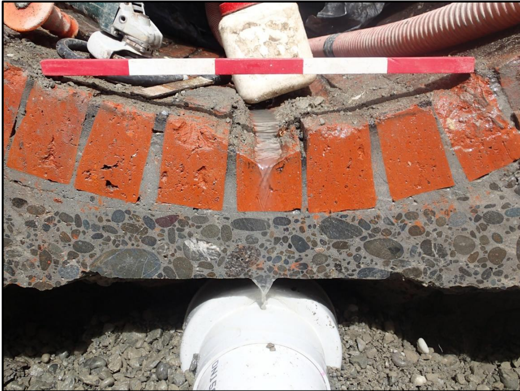
Figure 19. Detail of the invert at the eastern end of segment repair location 6. Note the groove formed in this brick, caused by the passage of grit and other particulate material washed into the sewer.
