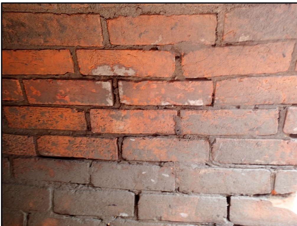
Figure 17. The inside of the brick barrel at the eastern end of segment repair 6, showing the arrangement of the bricks in a standard running bond.
