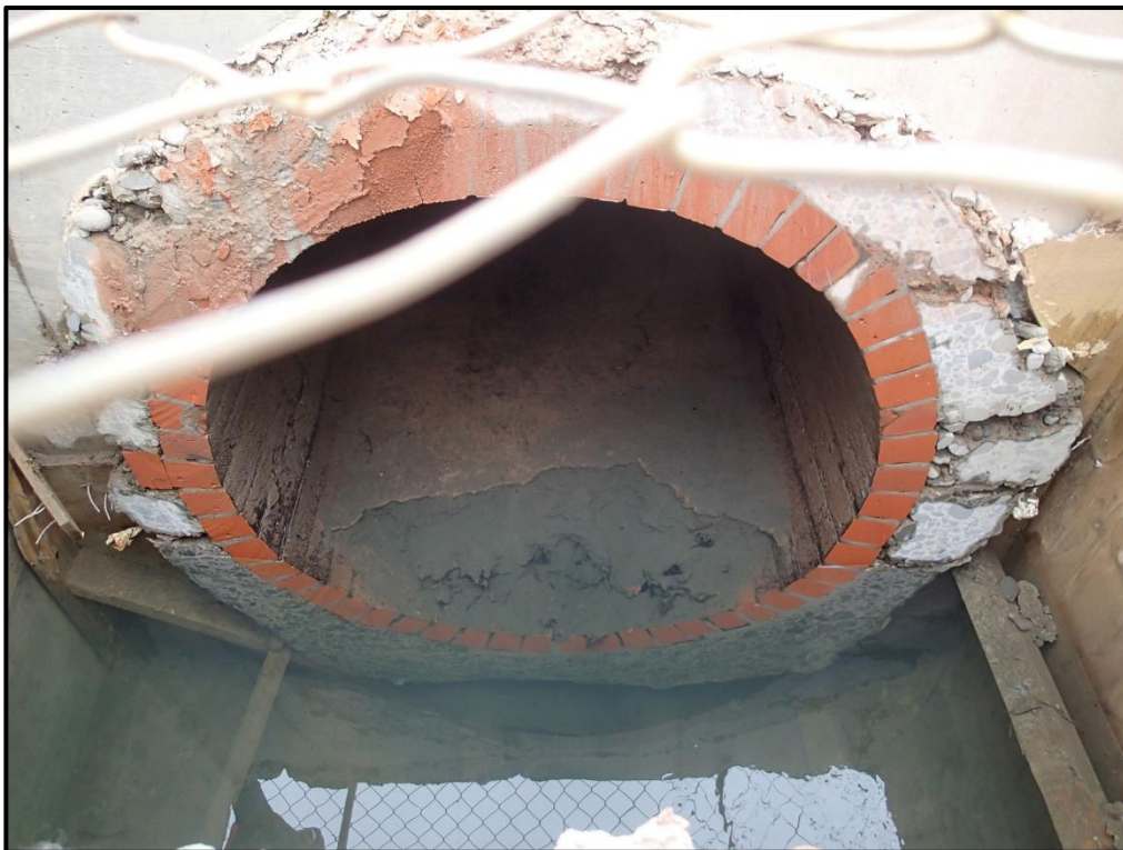
Figure 6. The eastern side of the brick barrel as exposed after wire cutting.
