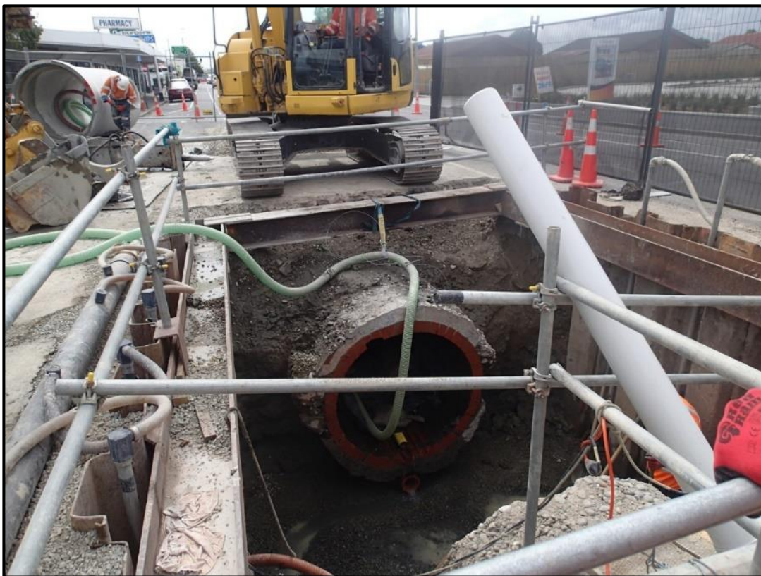
Figure 14. Looking northwest across the sheet-piled segment repair 6 excavation area.
