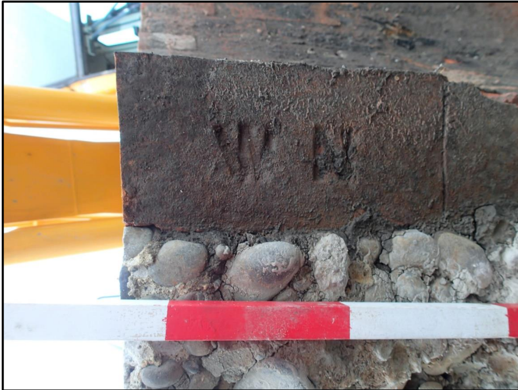
Figure 9. One of the marked 'WN' bricks used in the construction of the brick barrel.
