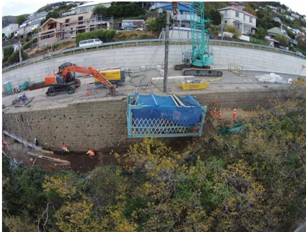
Figure 6: Soil nail getting inserted into Sumner Road retaining wall
