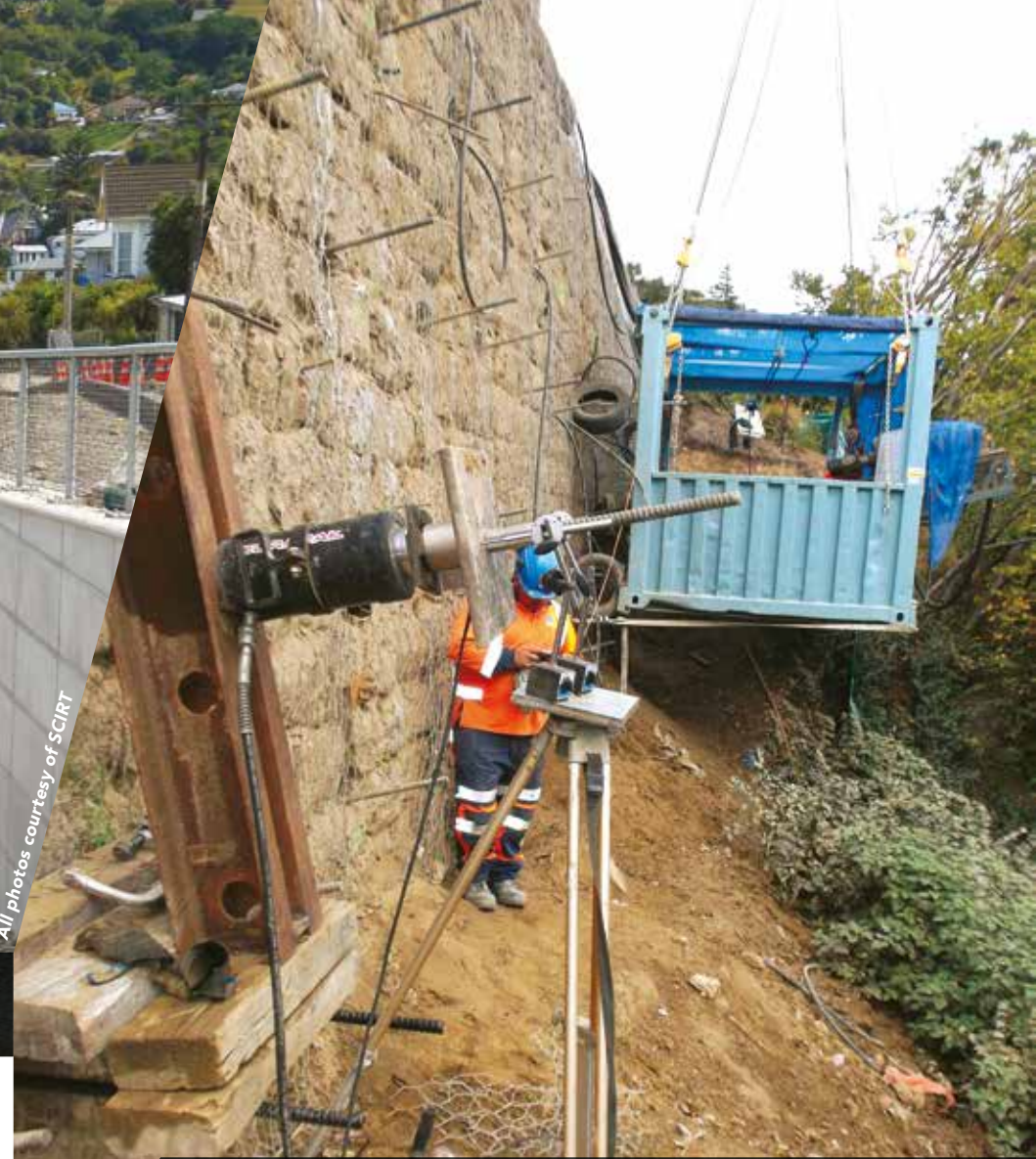
Testing the soil nails on stage four of the Sumner Road retaining wall repairs – a crane-suspended drilling platform was used to provide a safe working area
