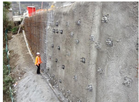
Figure 7: Engineer inspecting first layer of shotcrete
