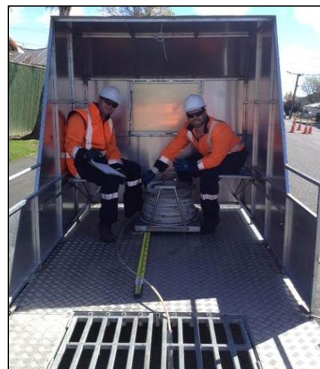
Trailblazers: An innovative pipe profilometer trailer boosts site safety.
