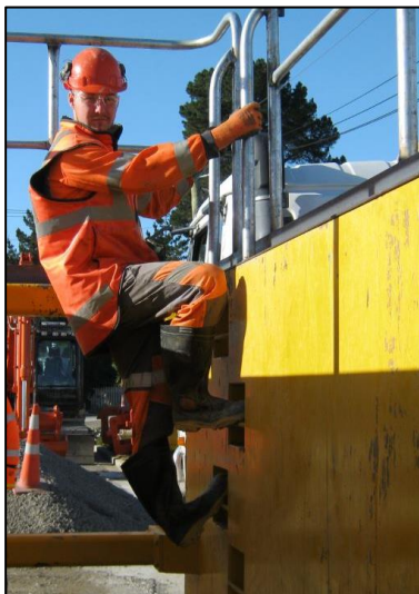
Protective shield: A worker uses trench safety railings.
