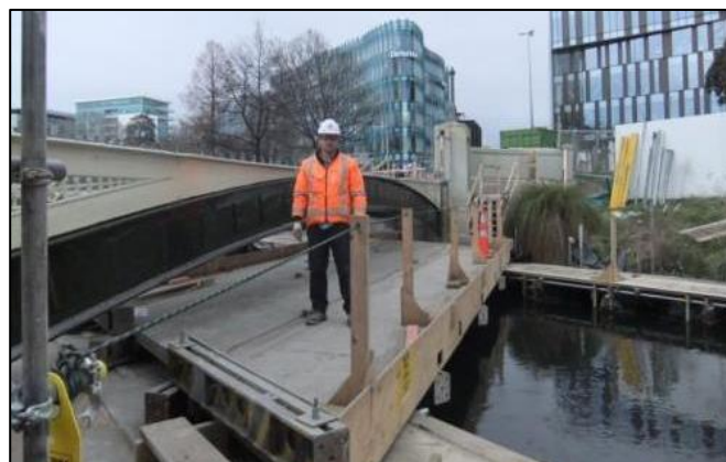
Bridging a need: A mobile work platform in operation at the Gloucester Street Bridge.
