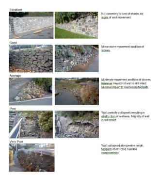
**Figure 3,** Example of condition rating for a stone facing wall.
