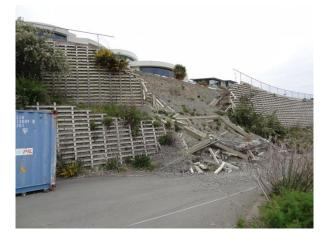
**Figure 1,** An example of earthquake related damage to retaining walls.
