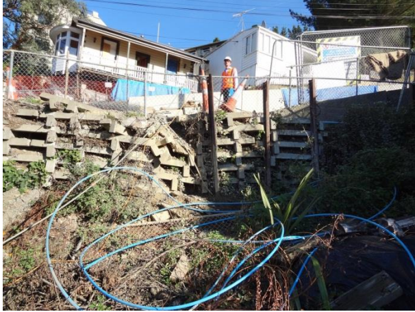
Figure 11. Damaged crib wall due for refurbishment as a soil nail wall
