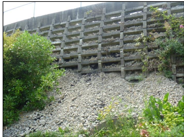
Figure 2. A crib wall showing bulging and loss of fill
