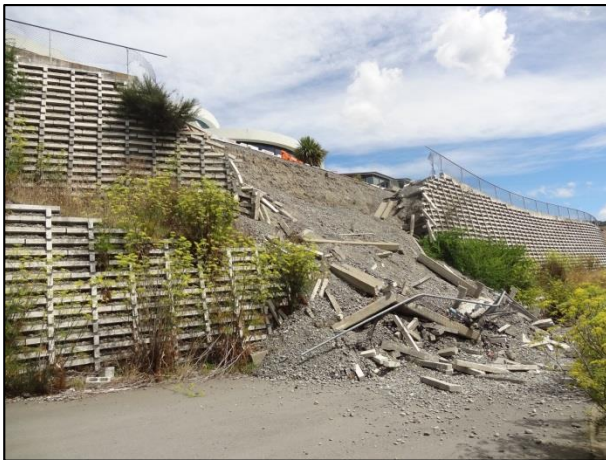
Figure 1. An example of a collapsed crib wall
