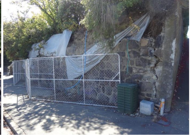
Figure 10. A partially collapsed stone wall showing typical damage
