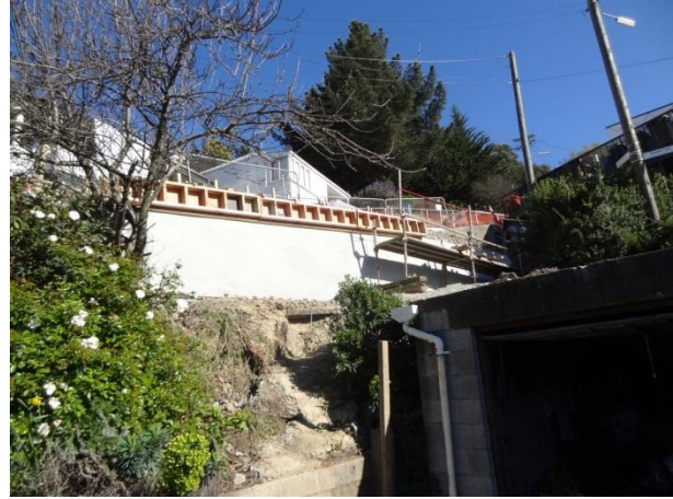
Figure 12. A soil nail wall refurbishment with shotcrete facing
