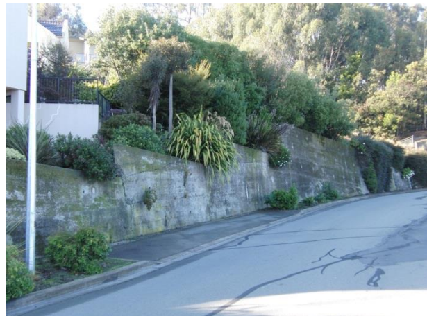
Figure 8. A concrete retaining wall c.1900 showing little damage
