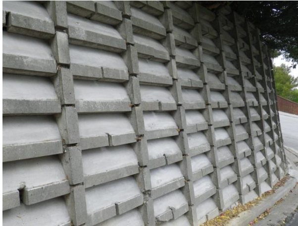
Figure 13. A crib wall with minor repairs to prevent future loss of fill
