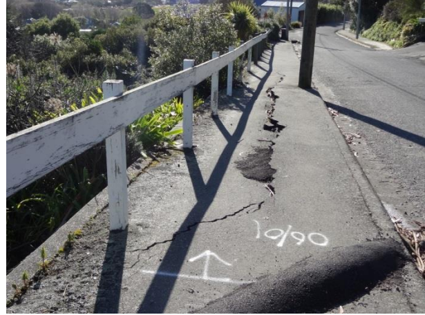
Figure 6. Footpath above a gabion wall showing cracking
