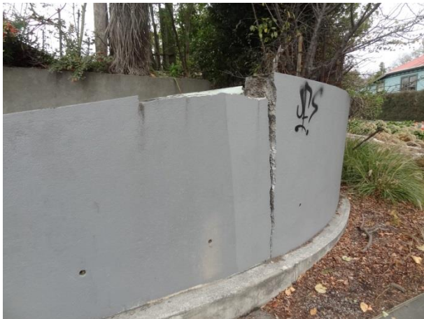
Figure 7. A typically damaged concrete retaining wall
