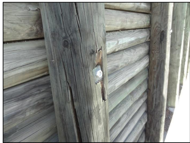
Figure 4. Damage around the anchor head of a timber pole wall
