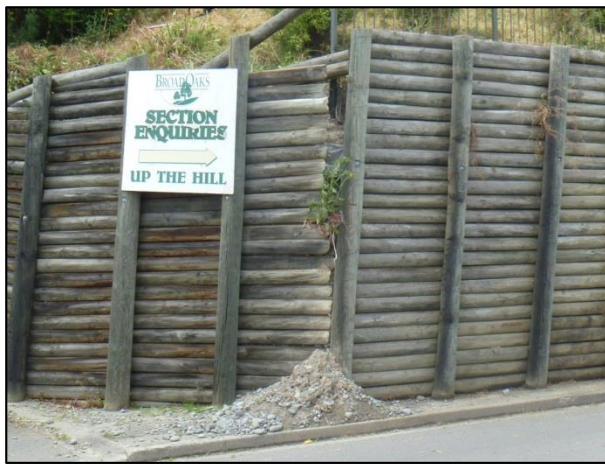
Figure 3. Damage to a vulnerable corner of a timber pole wall
