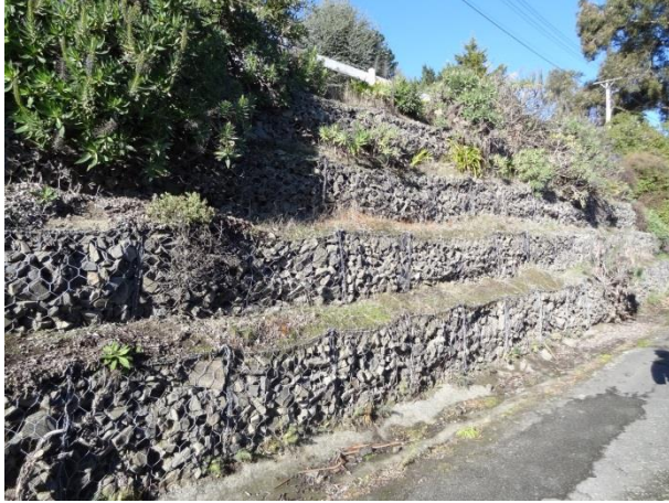
Figure 5. A badly deformed gabion wall
