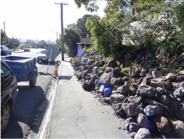
Figure 9. A completely collapsed stone wall
