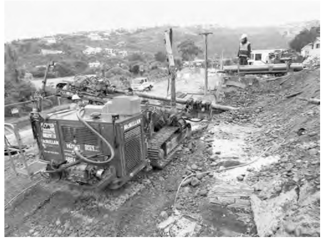
Photograph 7: Anchor Installation at Maffey's Road
