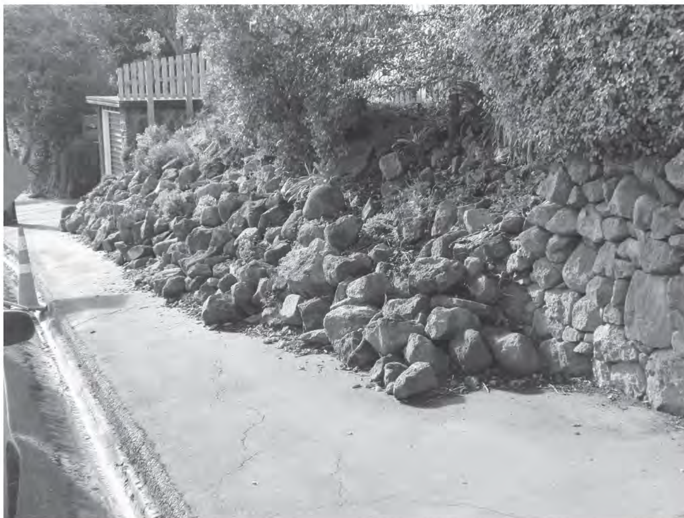
Photograph 1: Collapsed Stone Block Wall
