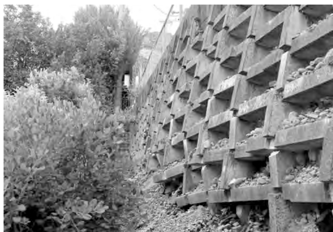
Photograph 3: Unvegetated Crib – fill loss and collapse.
