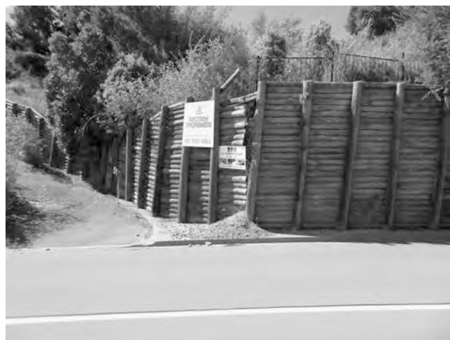
Photograph 5: Timber pole wall – damaged corner section
