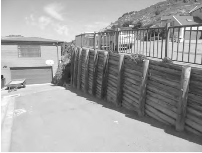
Photograph 6: Intact timber pole wall with cracked road behind
