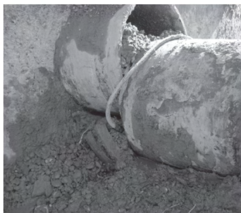
Photograph 11c: Damage to pipe connected to PS15 caisson
