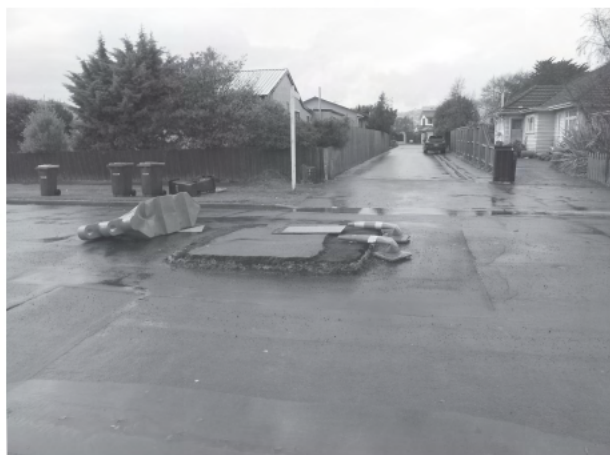
Photograph 11d: Floatation of manhole on street outside PS15
