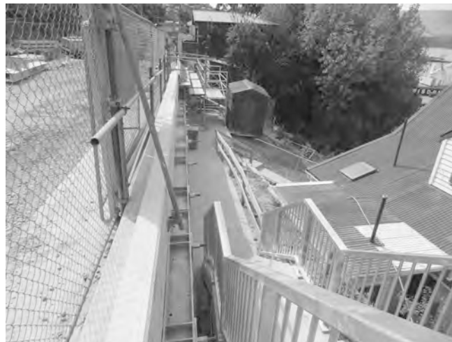
Photograph 10: Installed anchors and Waling at Cunningham Terrace
