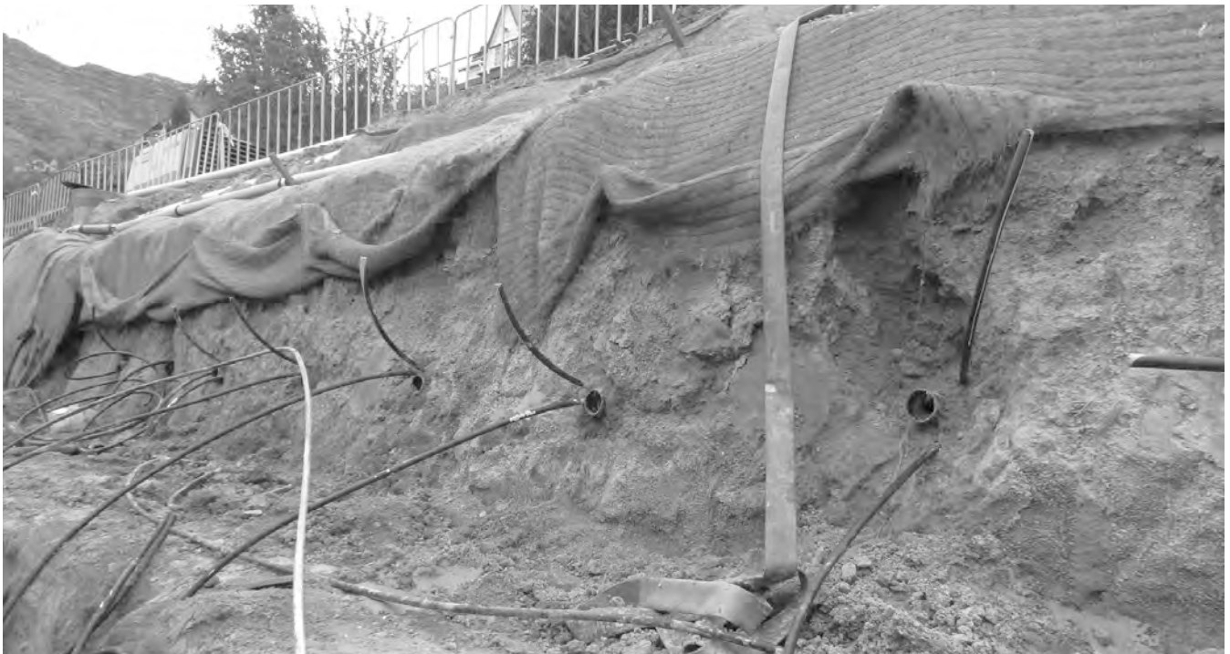
Photograph 8: Grouted Anchors at Cunningham Terrace
