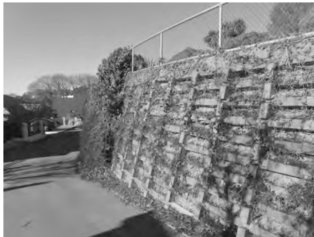
Photograph 4: Vegetated crib – fill intact & in good condition.
