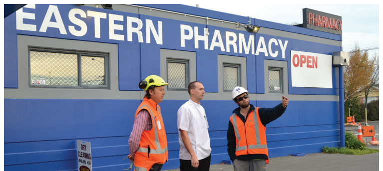
SCIRT staff discussing a pedestrian refuge with a business owner on Pages Road.
