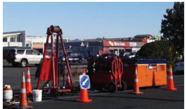
Pipe lining work sites generally take up less space than open trenching.
