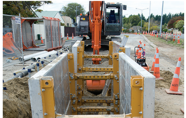
A typical trench being used to access services under the road.
