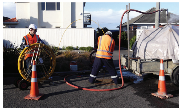
A pipe lining site. A cable and winch pull the pipe liner through the existing pipe from the manhole.
