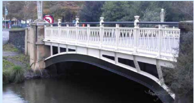
The reopened Colombo Street bridge, completed in April this year. Note the 'warping' on the right of the photo which was kept as an ongoing reminder of the February 2011 earthquake.
