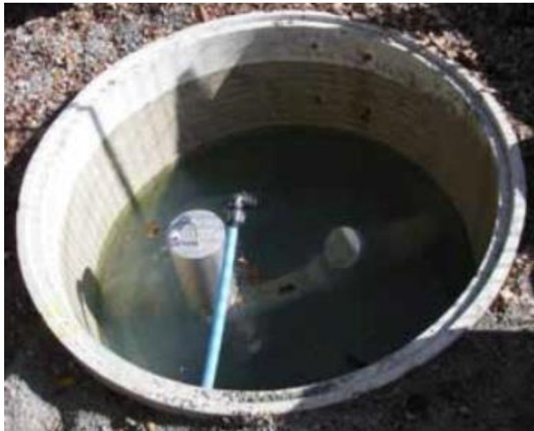
Figure 3: Steinhardt HydroFlush Device installed at Marley View Street
