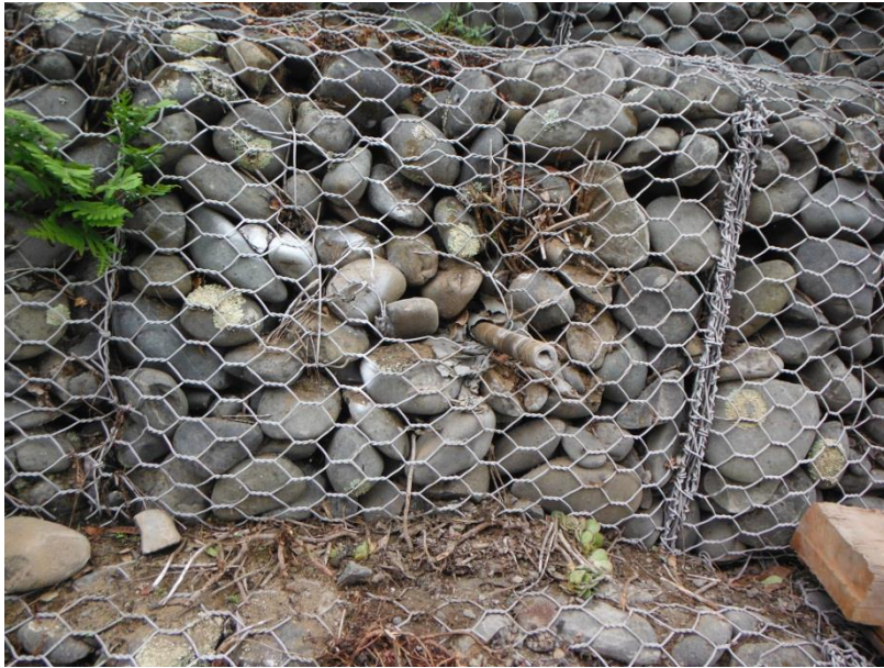
Figure 3 Resulting anchor head showing basket damage
