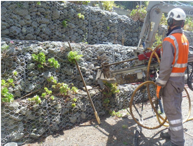
Figure 1 Anchor drilling through an existing gabion basket
