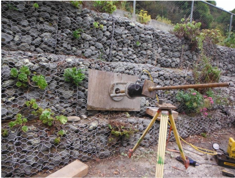
Figure 2 Anchor testing equipment
