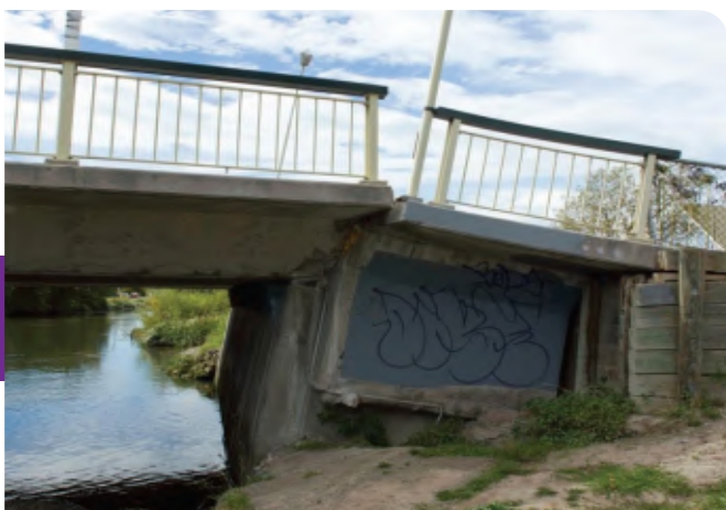
An example of how the ground has sunk near a section of the Avondale Bridge.
