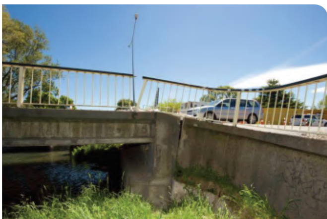
A damaged section of the Fitzgerald Avenue bridge over the Avon.
