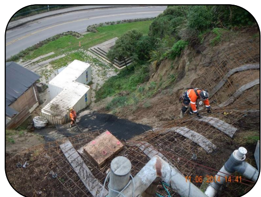
Drainage strips are installed to allow water to drain behind the concreted face of the retaining wall.
