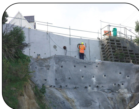
Crew member Sean McInerney connecting the storm water drainage.
