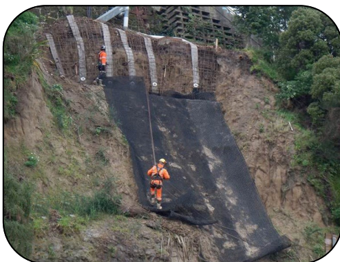
Reinforced geo-fabric is laid on the face of the slope to protect it from erosion.
