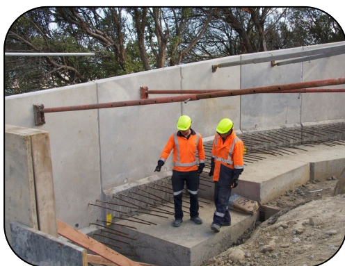
Jonathan Armstrong, Site Engineer, and Allen Costello, crew member, assessing the new concrete foundations of the retaining wall.
