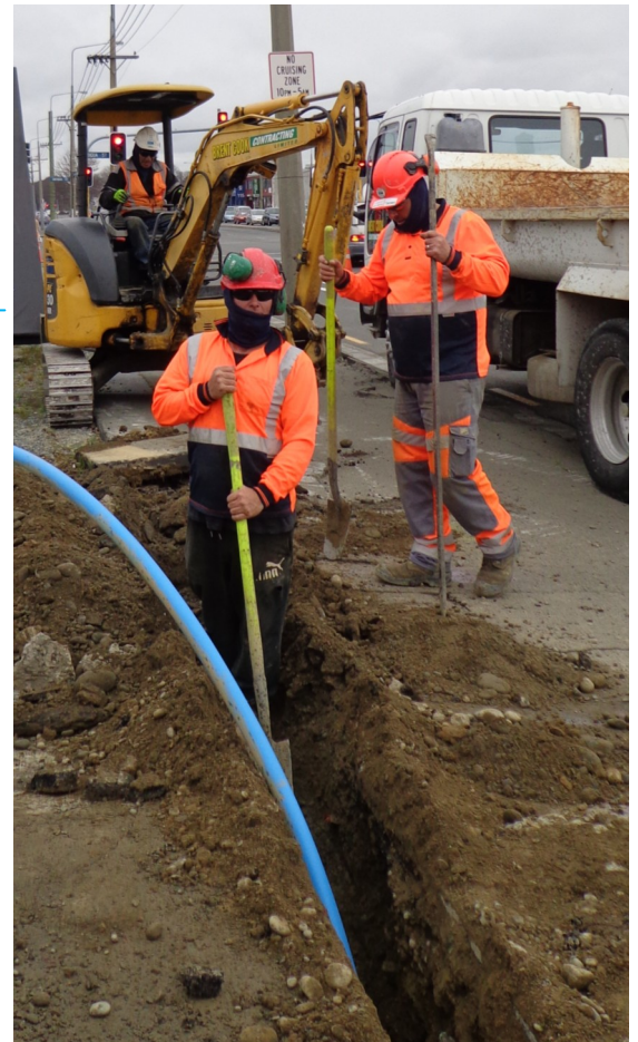
Picture 1. Open trenching the freshwater pipe in the footpath
