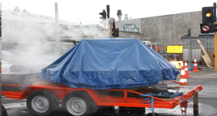
Heating the liner for the main wastewater pipe.
