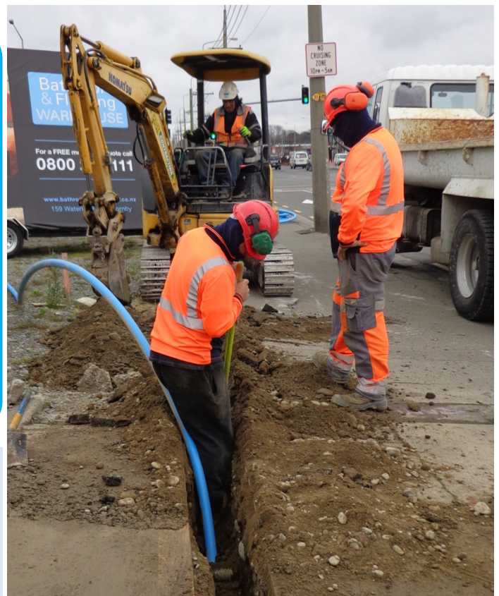
Replacing the freshwater sub-main pipe in the footpath
