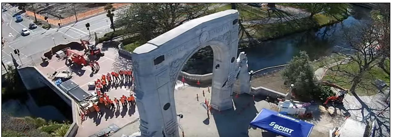
The restored Memorial Arch on the Bridge of Remembrance in Christchurch.
