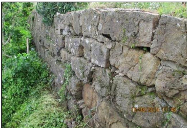
*Stress fracture: cracks in the wall of retaining structures.*
