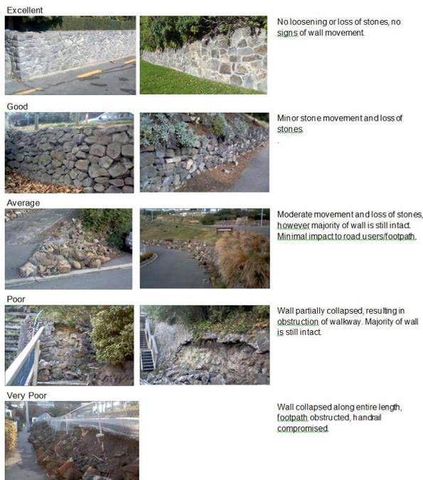
**Figure 3**, Example of condition rating for a stone facing wall.
