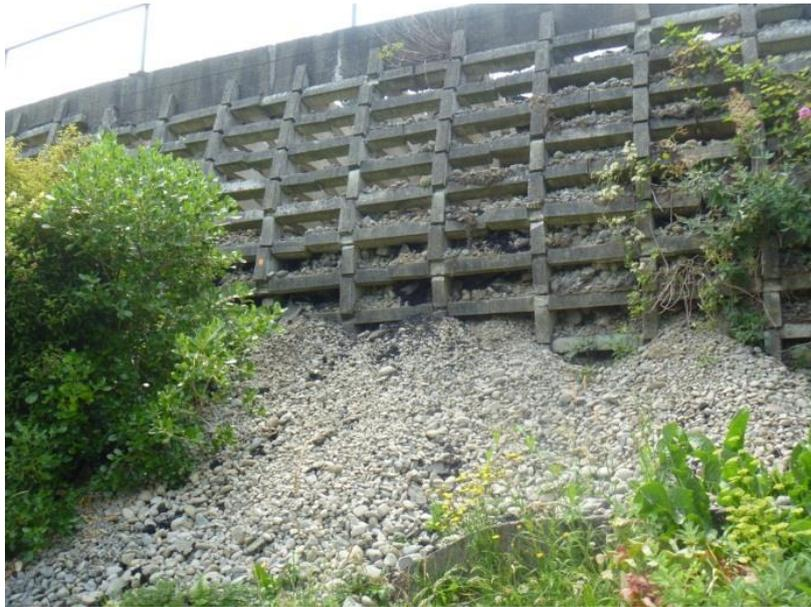
Figure 1 The damaged Cunningham Terrace retaining wall
