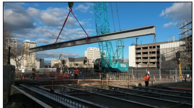
Beam up: A section of the Gloucester Street Bridge is hoisted into place
