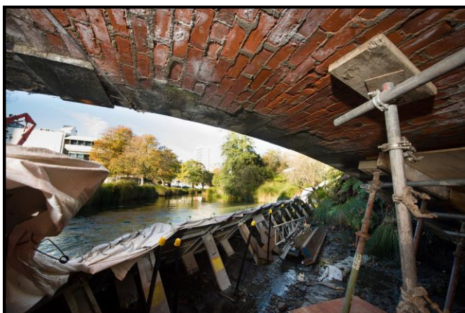
Brick by brick: Work gets underway on the Armagh Street Bridge.
